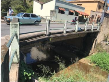
Ponte – 11,0 x 4,5m
