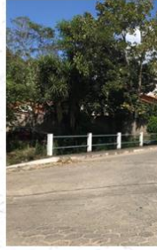
Ponte – 9,00 x 4,50m
