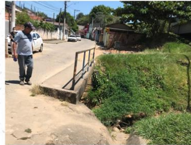
Ponte – 7,20 x 3,10m
