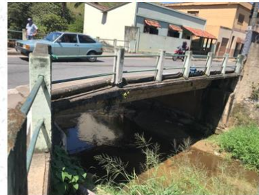
Ponte - 11,0 x 4,5m
