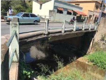
Ponte - 11,0 x 4,5m
