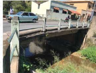
Ponte - 11,0 x 4,5m
