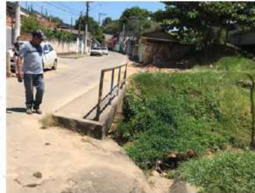
Ponte - 7,20 x 3,10m
